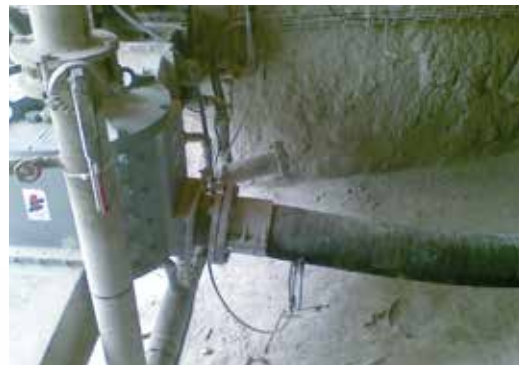
Micro-silica conveying 1 silo feeds 5 separate lines.
